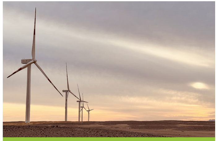
Photo: Courtesy of West Bakr wind farm
